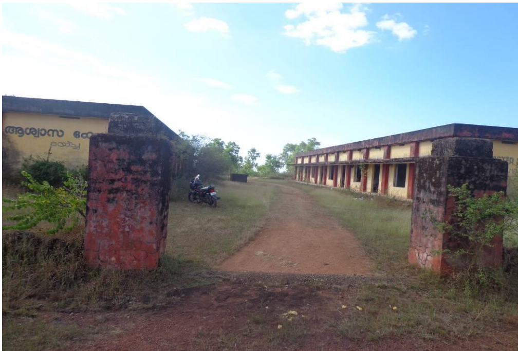
3 and 4: View of the site. Dilapidated Shelter in the site can be seen
