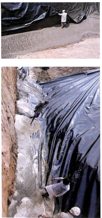
The LDPE sheet is being lowered into the trench before its anchoring into the PCC layer.
