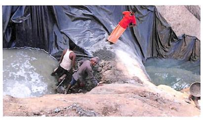
Embedding the LDPE sheet in the sector where the rock is exposed as a barrier in the trench.
