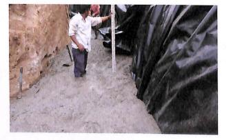
The trench being manually cleaned such that all debris and mud are removed. The fresh rock- migmatite- is exposed in the trench.
