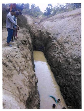
View of the trench looking south from the northern edge. Partly weathered rock is exposed in the trench. Fractures are visible. The presence of a hard rock barrier in the centre of the trench has limited the progress of excavation. Workers are in action to ensure that continuous dewatering is carried out and the water level does not rise.
