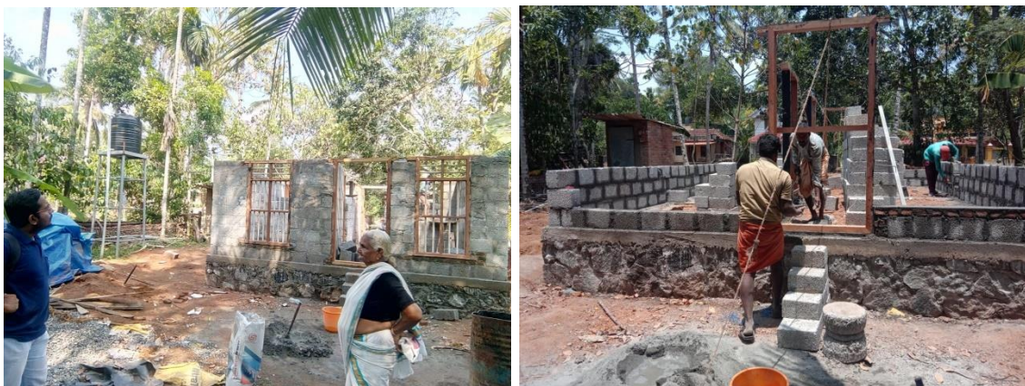
Lakshmikuttyamma's House Under Construction
