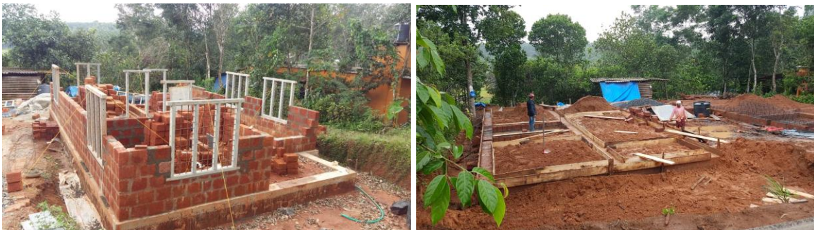
Praveen's And Unnikrishnan's House Construction
