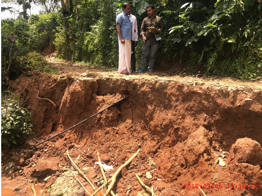
Figure A-5: Landslide scarp @ 9.7968694° N 77.0675658° E
