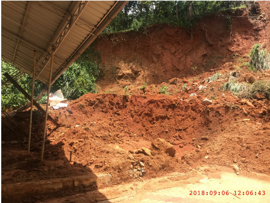
Figure A-3: Landslide near a gas station @ 9.8549653° N 76.9619187° E
