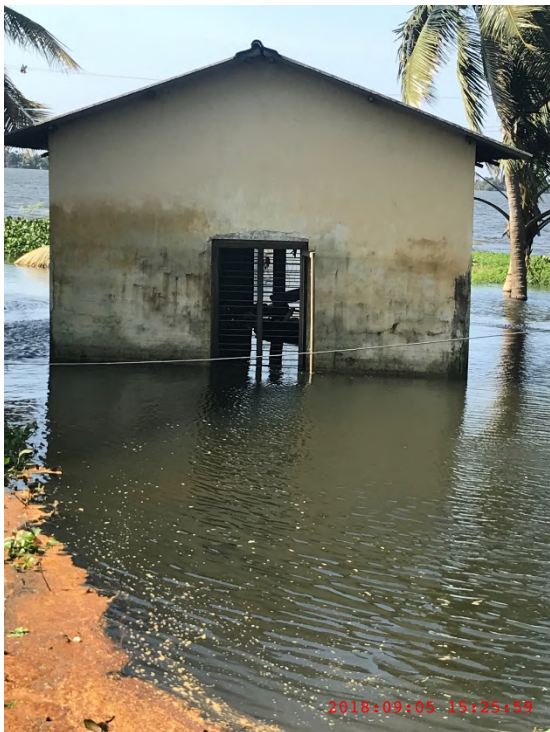
Figure 5.9: Flooded home due to bund failure @ 9.5032691°N 76.3776221°E
