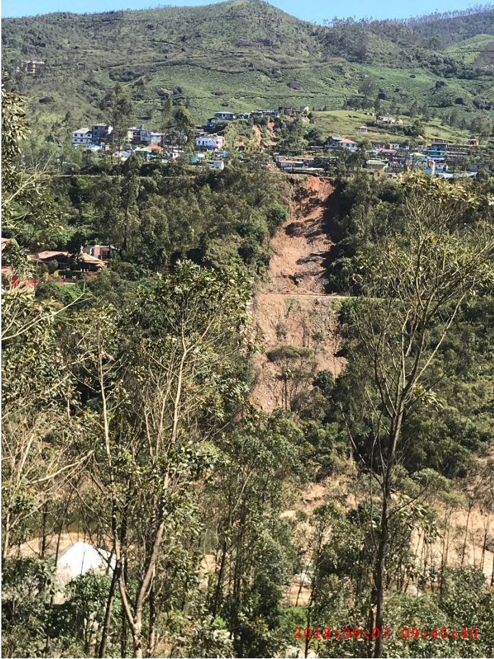
Figure A-15: Debris flow failure @ 10.0830840° N 77.0711627° E
