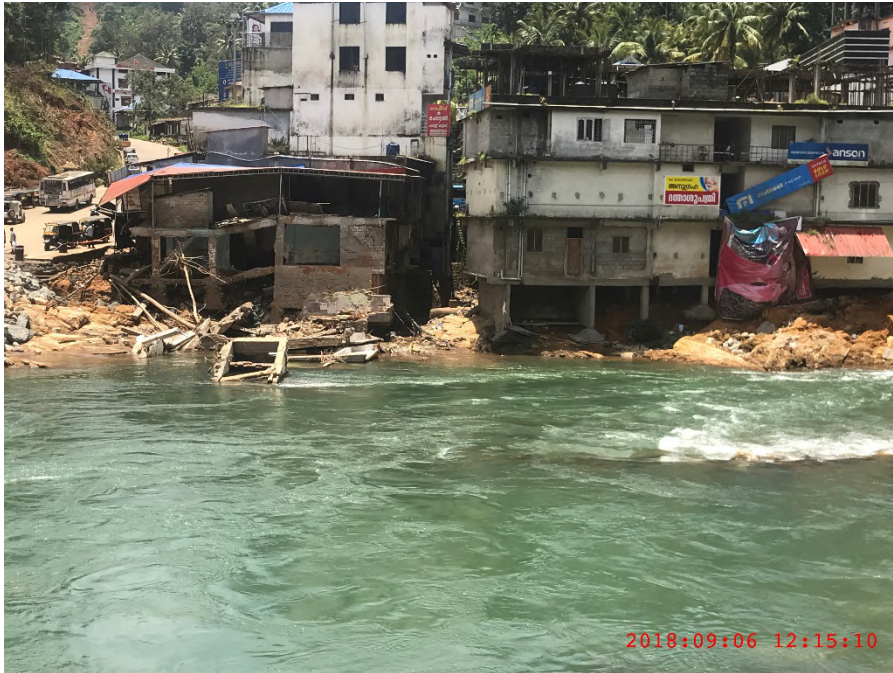
Figure B-2: River erosion @ 9.8575868^{\circ} N 76.9636007^{\circ} E
