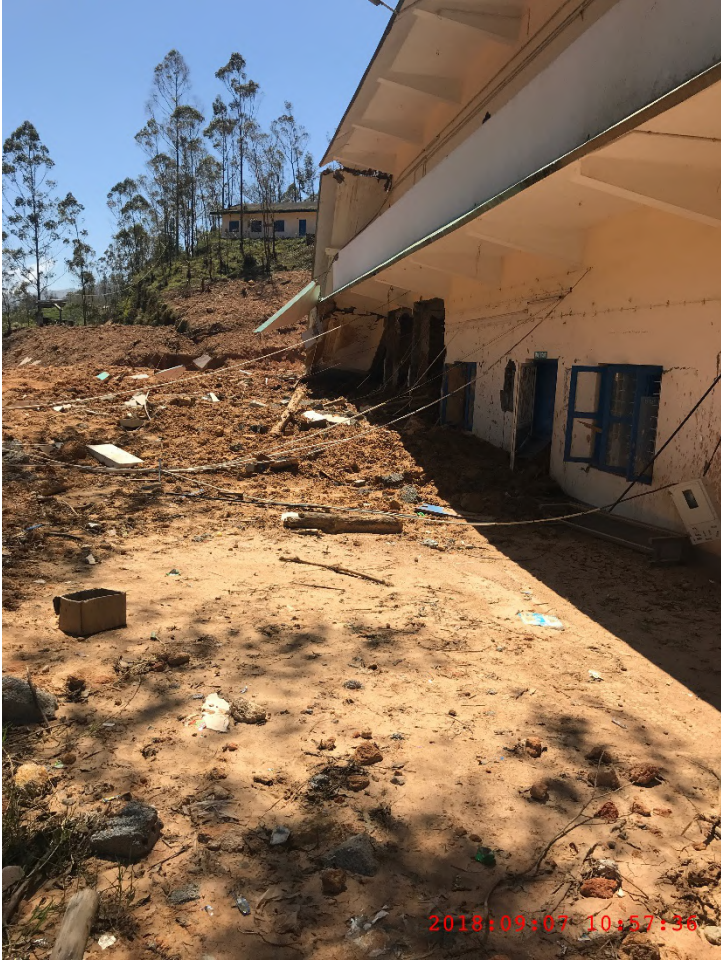
Figure A-18: Destroyed Munnar College building @ 10.0826962° N 77.0726538° E
