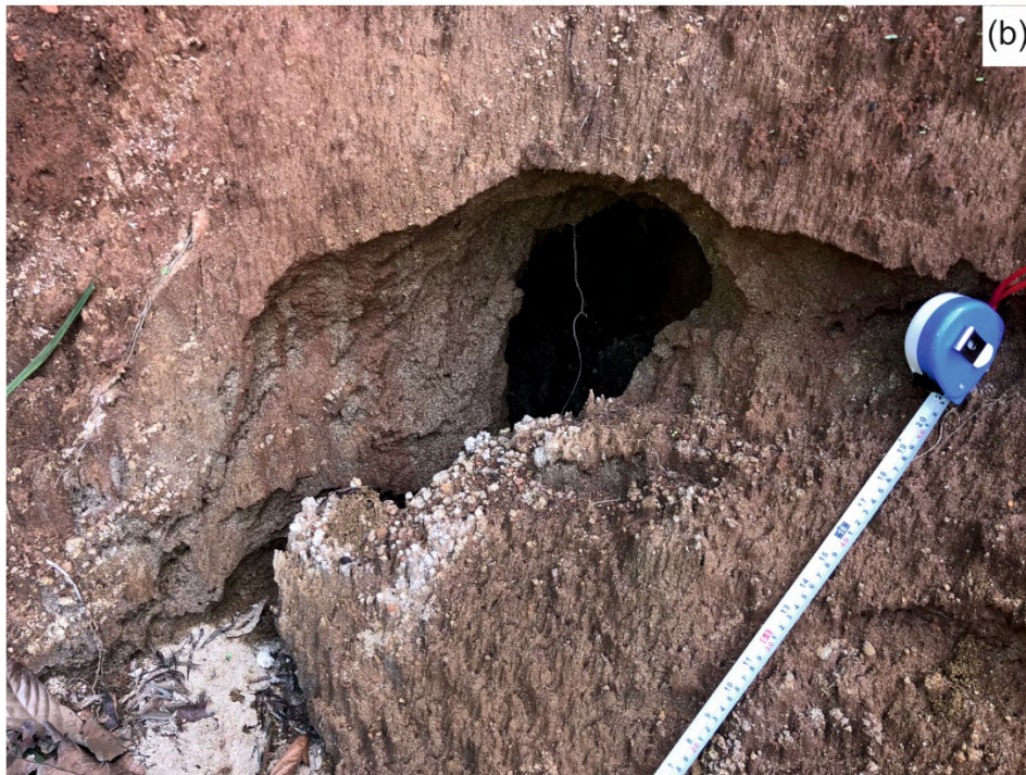
Figure 2.8 (a) Landslide at Vellathooval (b) Surface manifestation of a conduit in piping phenomena 10.0088136°N; 77.0257626°E
