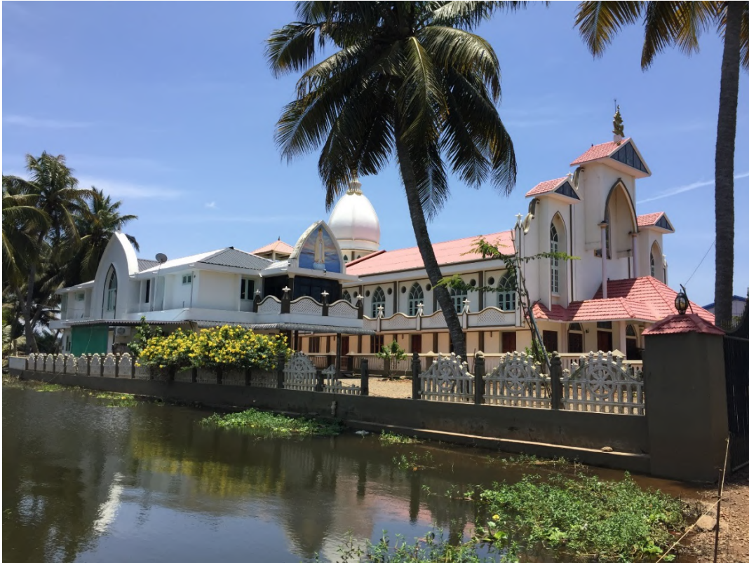
Figure 4.11: Mar Sleeva Church. Original Church constructed on 30-foot long concrete piles; ancillary building constructed on six- to eight-foot long sections of coconut trees placed in nine-pile groups (Latitude=9.450352°, Longitude=76.389449°).
