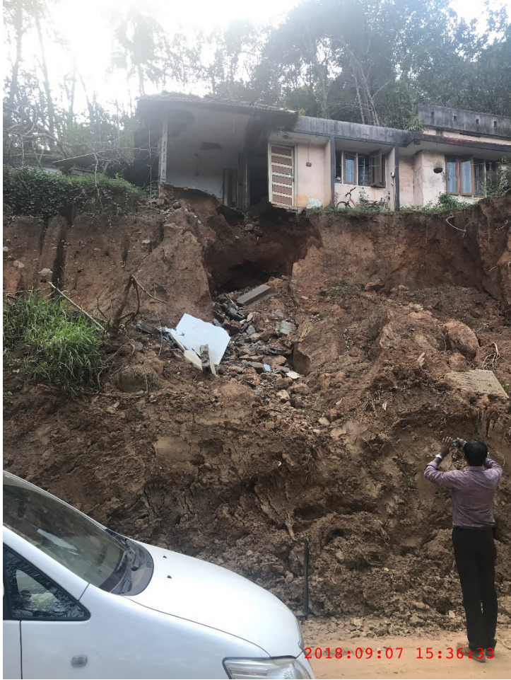
Figure A-24: Another view of the pipping channel @ 9.9756741^{\circ} N 77.0216901^{\circ} E
