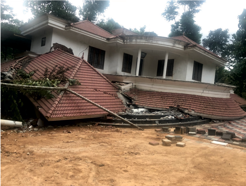
Figure 2.3: Collapse and submergence of one storey near Mavadi 9.8747275°N; 77.1194017°E.
