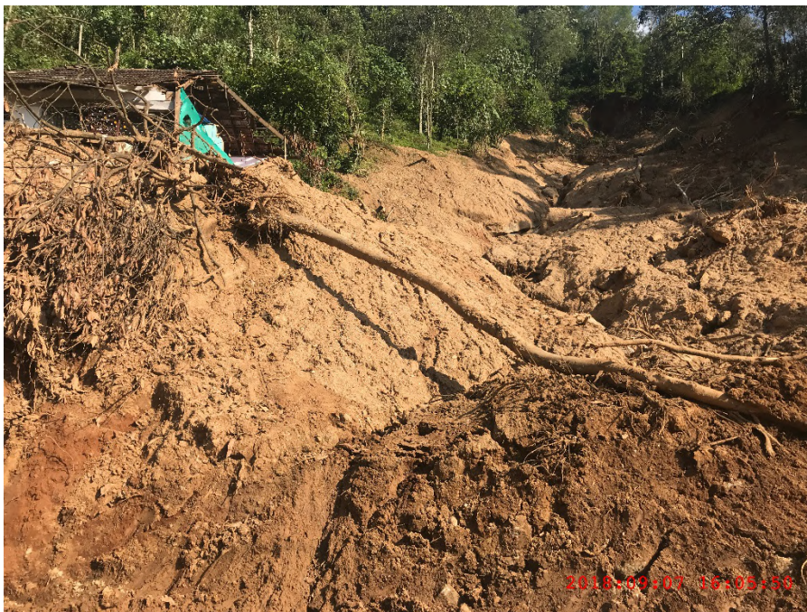
Figure A-28: Seen on the left is a house that has been destroyed in Panniyarkutty landslide @ 9.9748956° N 77.0427662° E
