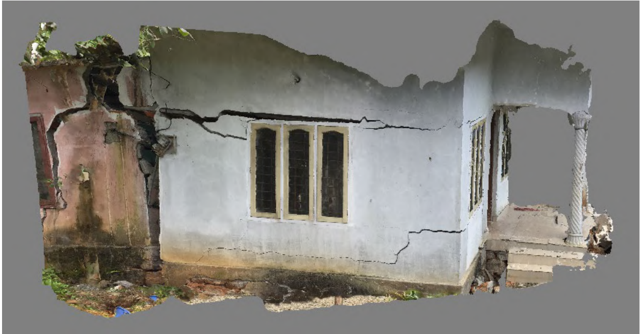
Figure 2.17: Left side isometric projection of the three-dimensional reconstruction of one of the houses within the Idukki Landslide by means of Photoscan (9.7962622°N; 77.0681814°E).
