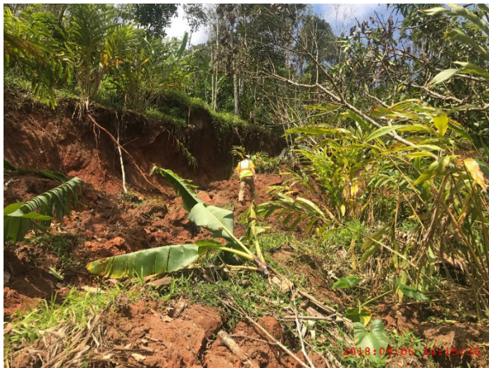
Figure A-10: Landslide scarp @ 9.7970015^{\circ} N 77.0683650^{\circ} E
