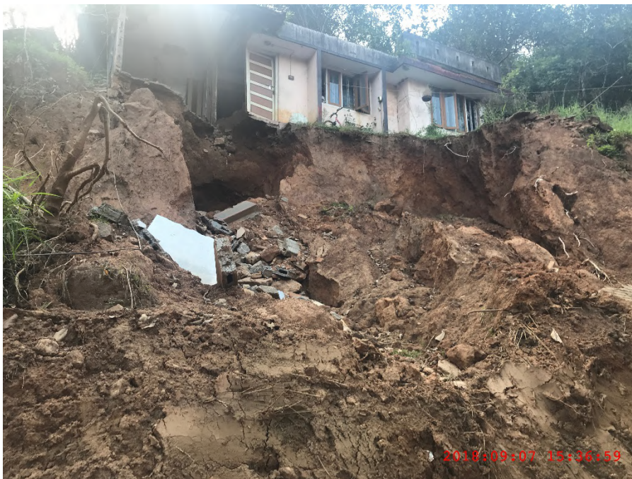
Figure A-23: A landslide case with large pipping channel @ 9.9756943^{\circ} N 77.0216695^{\circ} E
