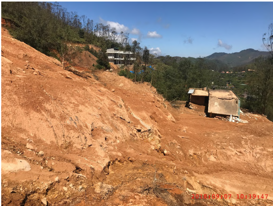
Figure A-17: Munnar college landslide showing the destroyed college building @ 10.0822577° N 77.0734317° E
