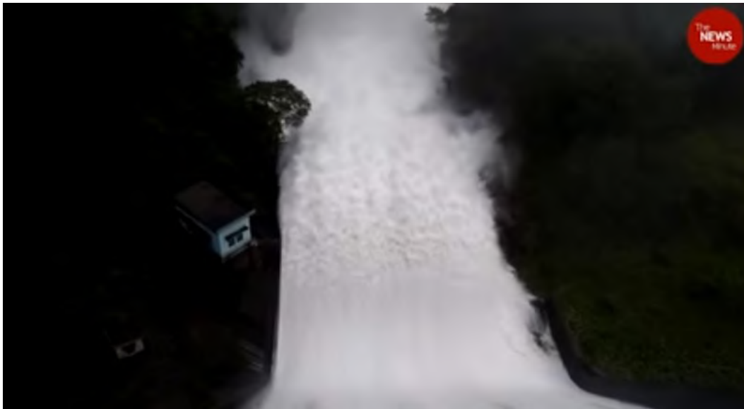
Figure 3.3: Shutters of Idamalayar dam in Kerala opened as reservoir hits full capacity source: The News Minute
