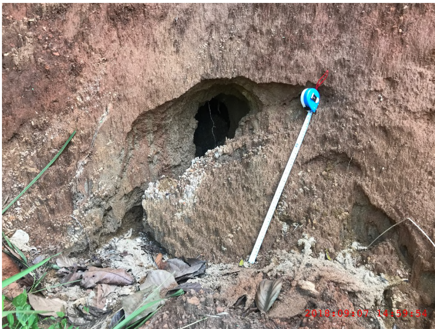
Figure A-21: Another view of the pipping @ 10.0088132^{\circ} N 77.0257597^{\circ} E
