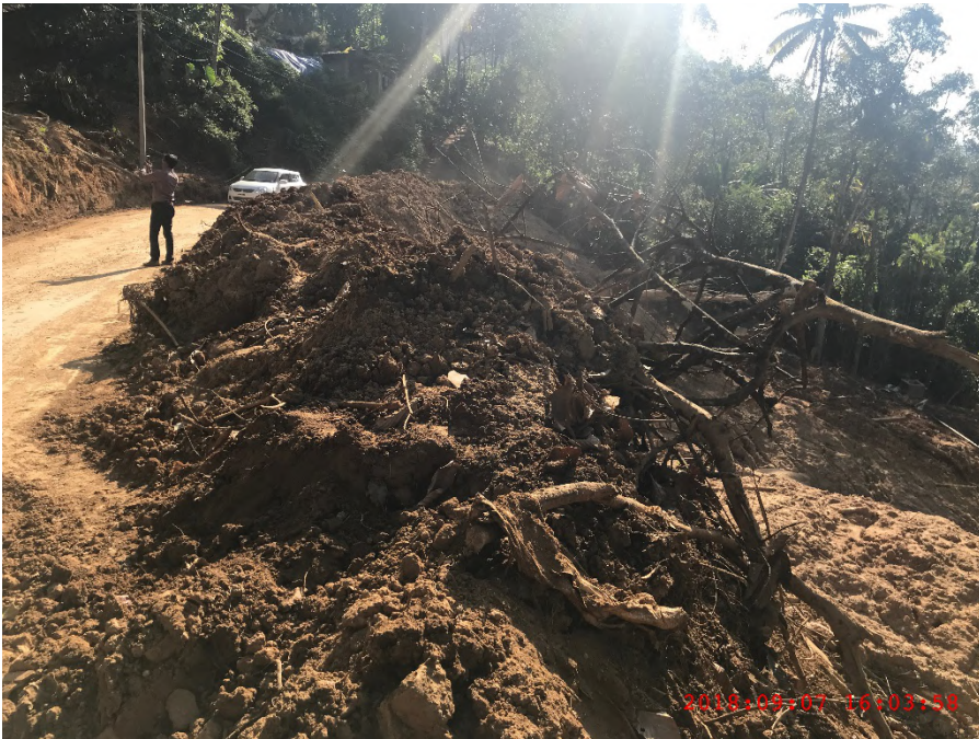
Figure A-26: Panniyarkutty landslide @ 9.9749966° N 77.0429146° E
