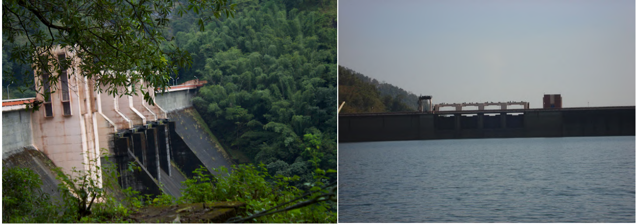
Figure 3.2: Downstream and upstream view of the Idamalayar dam. Source Wikipedia contributors, 2018)
