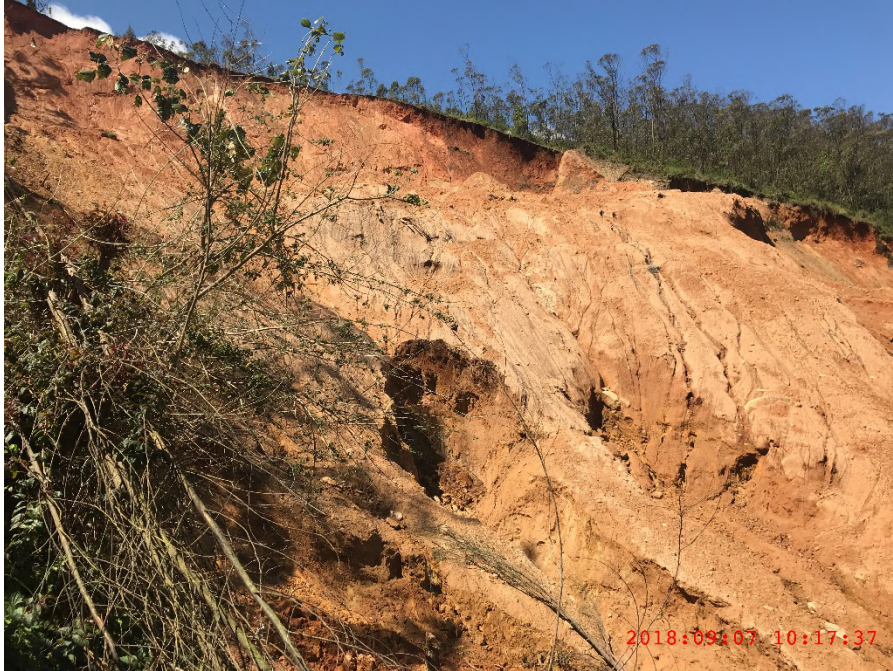
Figure A-16: Munnar college landslide showing piping channels @ 10.0822483° N 77.0734512° E
