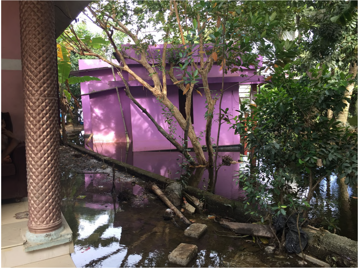
Figure 4.1: Photograph of the subsided purple house located at coordinates Latitude=9.4626°, Longitude=76.3659°.
