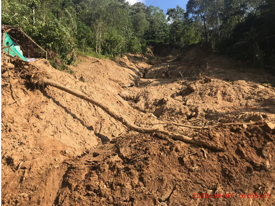
Figure A-27: Origin of the Panniyarkutty landslide @ 9.9748956° N 77.0427662° E
