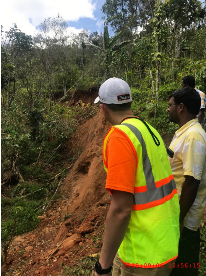
Figure A-9: Landslide scarp @ 9.7966110^{\circ} N 77.0685257^{\circ} E
