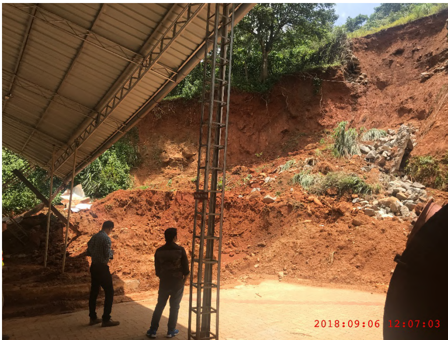
Figure A-4: Landslide near a gas station @ 9.8549653° N 76.9619187° E
