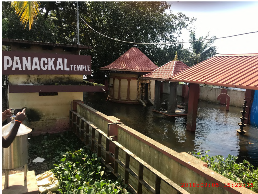
Figure 5.6: Flooded temple complex from the bund failure @ 9.5033596°N 76.3771085°E
