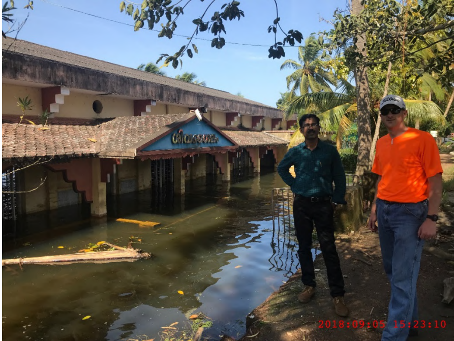
Figure 5.8: Entrance of the flooded community hall @ 9.5033389°N 76.3772861°E
