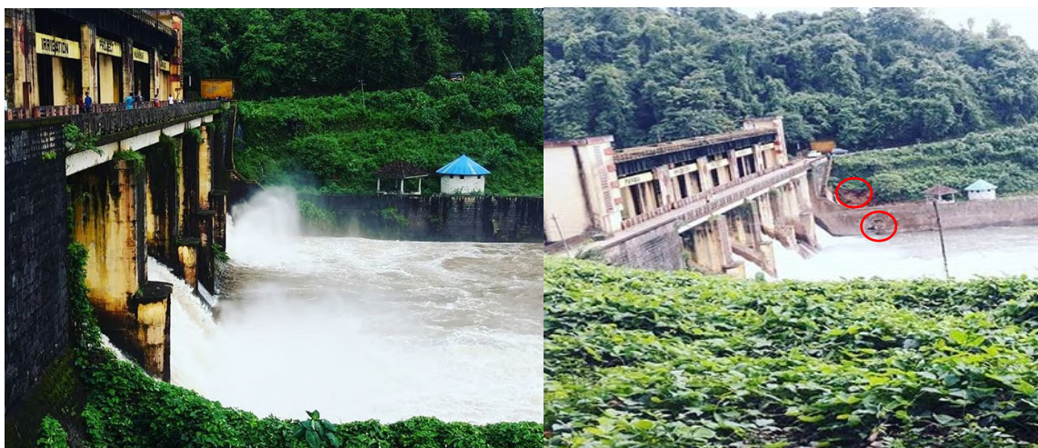
Figure 3.8: (Left) Downstream side of the Maniyar Dam with the shutters open on August 10th. (Right) Similar view as the left image taken on August 25 th showing minor slope failure and damage to the retaining structure (failures are circled in red). Source of photograph: Instagram
