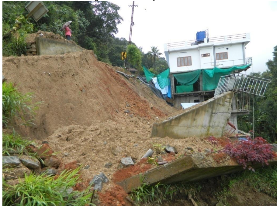
Fig: Accumulated remains of building and debris.
