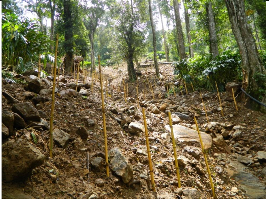
Fig: The upper part of the failed surface.
