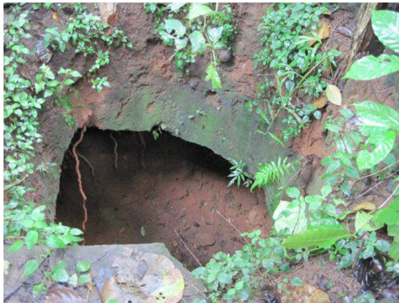
Figure 3.40: opening of a subsurface tunnel within the well
