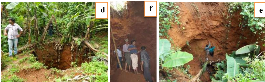
Figure 3.24: Unstable Soilpipes in Kottathalachimala, Kannur
