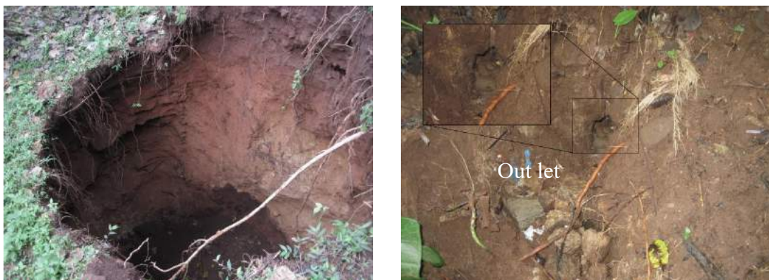
Figure 3.42: Inlet and outlet of Piping in Nalaam mile, Idukki district
