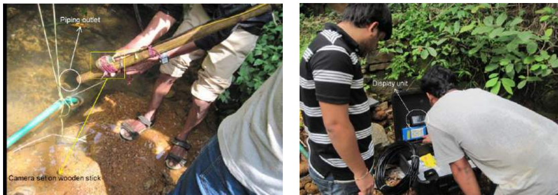
Figure4.39 Using of push camera inside the Tunnel in Chattivayal, Kannur
