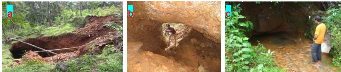
a. Piping Inlet, b. Middle opening of pipe, c. Piping Outlet
