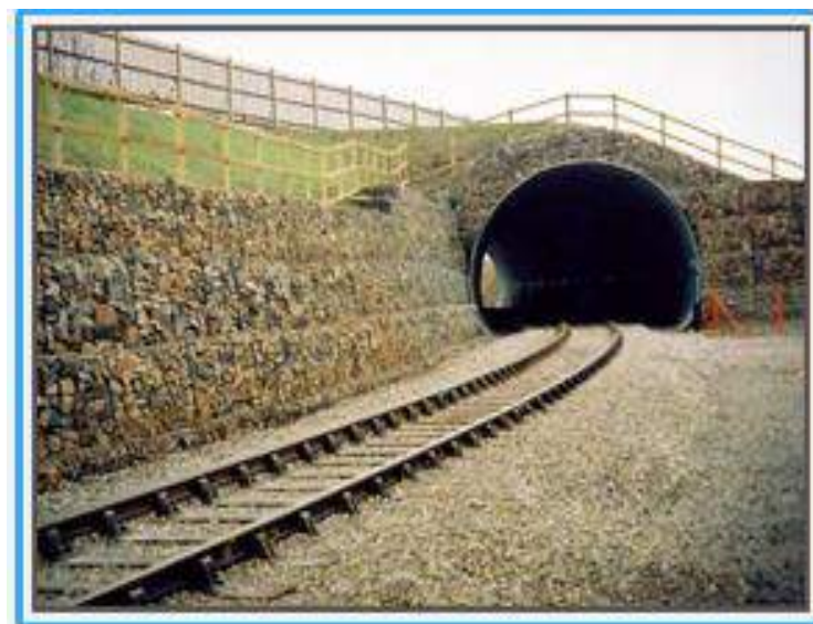
Figure 7.7 Gabions along railway tracks (Panjami 2016)
