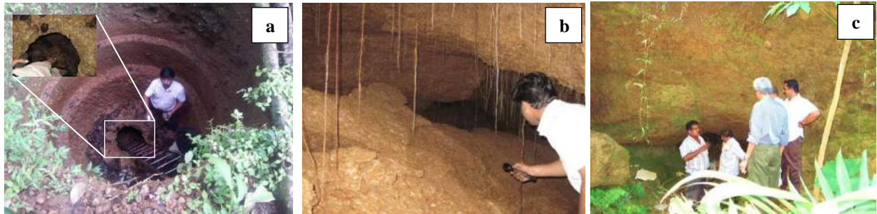
Figure: 3.29 Soilpiping affected well at Niranganpara, Kannur
