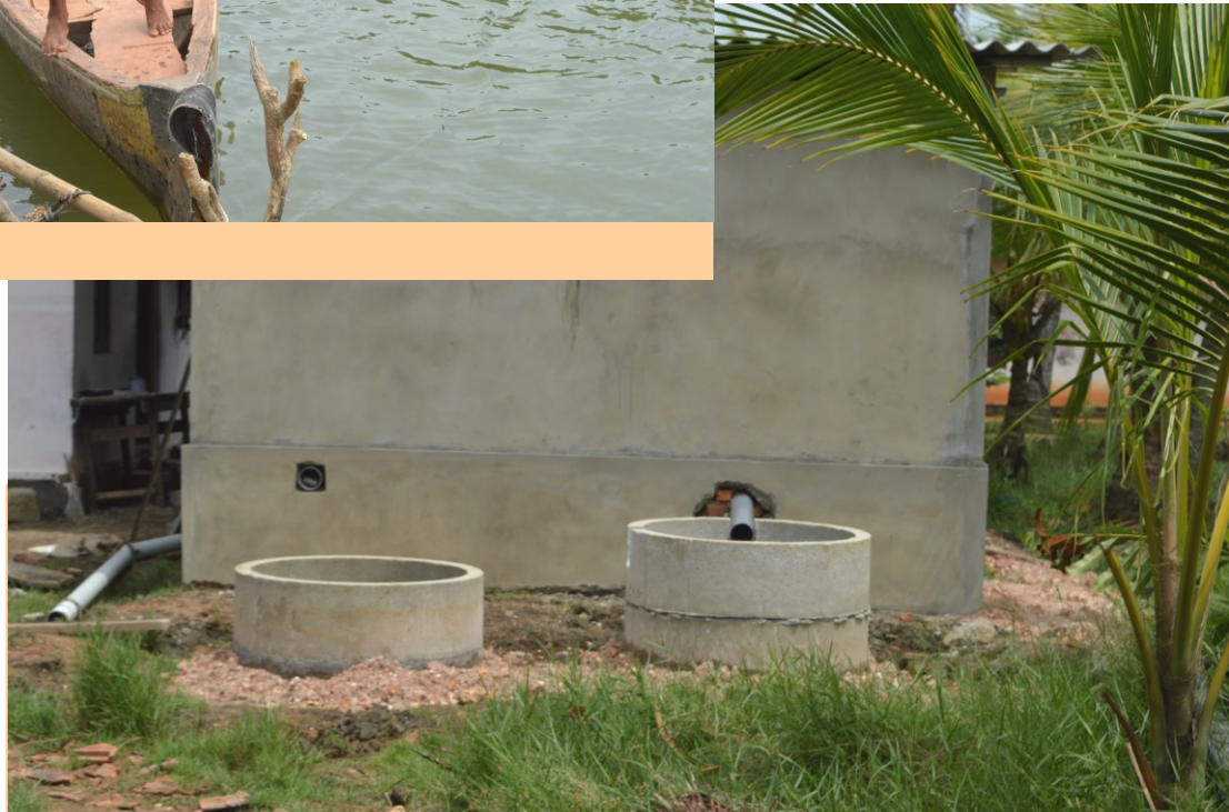
Pit Latrine under construction
