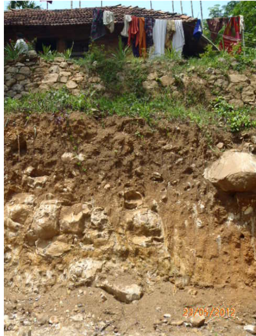
Figure 3: Entrapped boulders and cobbles in the B & C horizons
