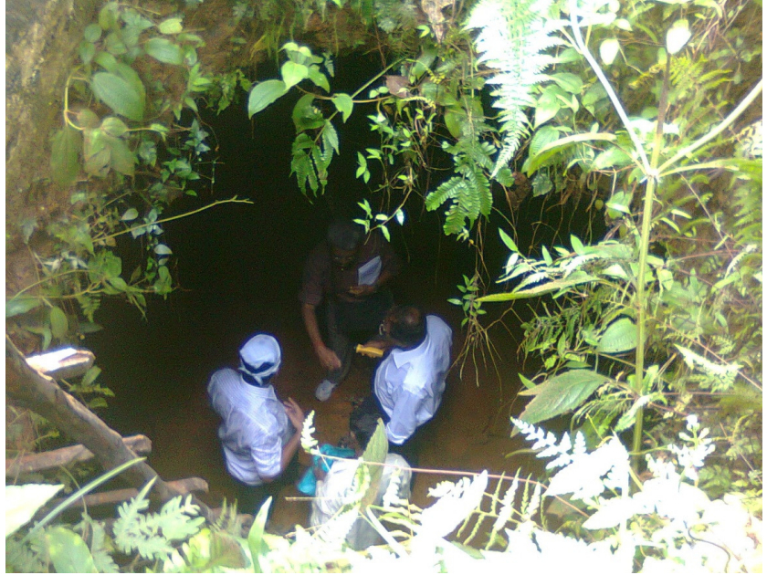
Figure 2: Inside the pipe in Mr. Bhasi's property
