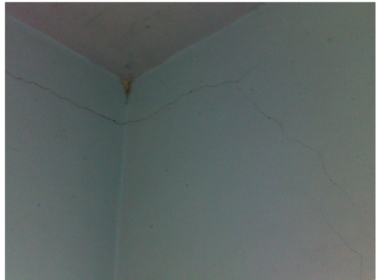
Photographs of cracks developed over masonry structures during the earthquake
