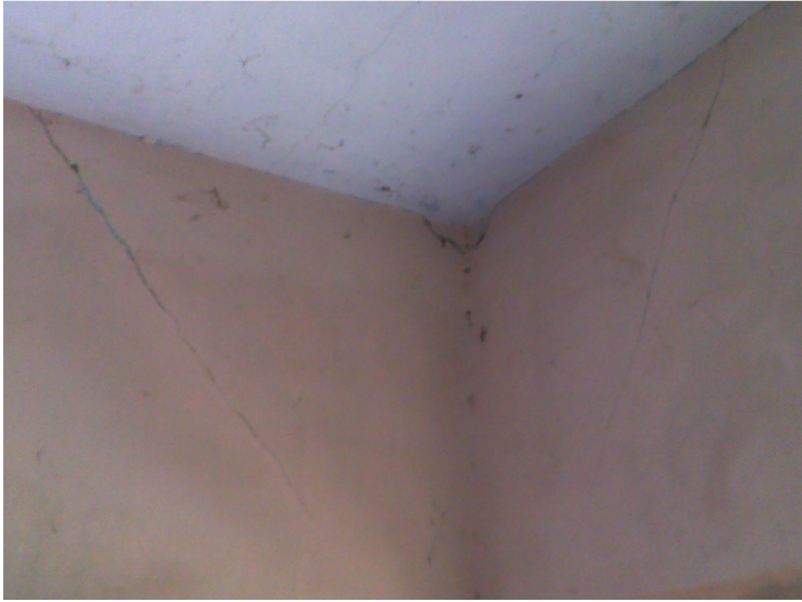
Photographs of cracks developed over masonry structures during the earthquake
