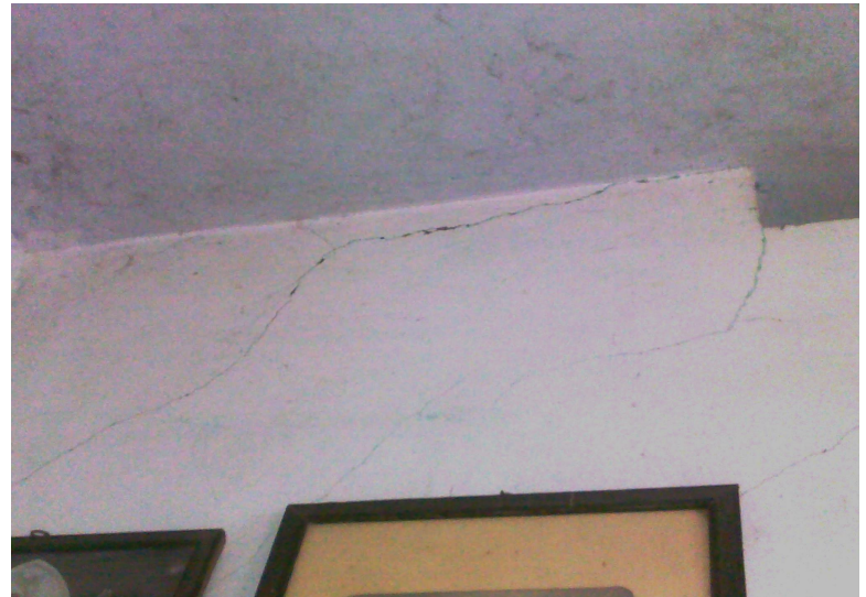
Photographs of cracks developed over masonry structures during the earthquake
