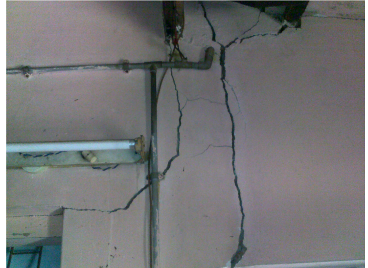
Photographs of cracks developed over masonry structures during the earthquake
