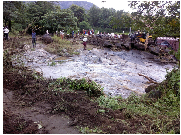
Figure 12: Photograph of the railway track affected by landslide. Note the large tree trunks brought from the upper slopes. The wagons in still in supported condition.
