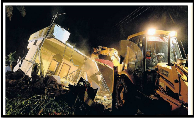
Building collapse due to heavy rain at Aluva, Ernakulam 07.08.2014
