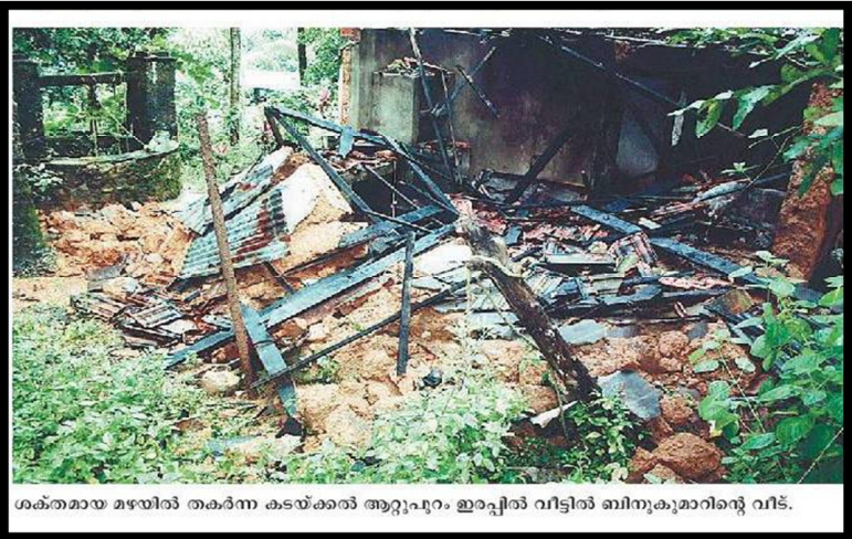
House damage at Kadakkal Aattupuram, Kollam 24.08.2014
