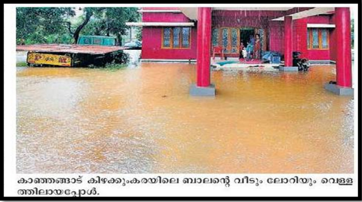
Flooded house due heavy rain at Kanhangad, Kasaragod 02.08.2014
