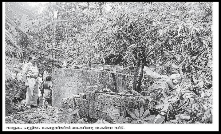
House damages at Valakam-Puliyam colony Kottarakkara, Kollam 20.06.2014
